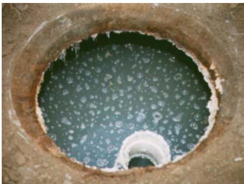
Pictured is a septic tank that had not been pumped for over three years. Normally floating sludge over an inch thick would be present. The tank was only treated for one year with 1 lb. of Ultra-Archaea every month. There is very little bottom sludge. The bubbles floating on the top are soap suds. The effluent leaving the septic tank is clear indicating that the septic tank is functioning properly.
